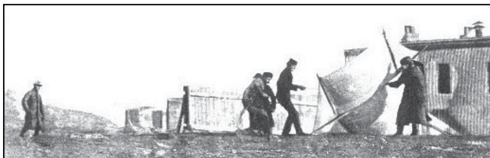
Photograph of Marconi and associates raising the receiving antenna by kite at St. John's, Newfoundland in December, 1901. Appeared in the article "Marconi's Achievement" in the February, 1902 issue of McClure's Magazine
